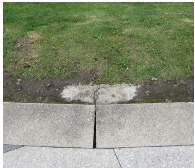
Image below: Example of topsoil washout. The haunching is set near the top of kerb allowing for minimal topsoil to be placed, therefore prone to erosion over time. Credit KCC
