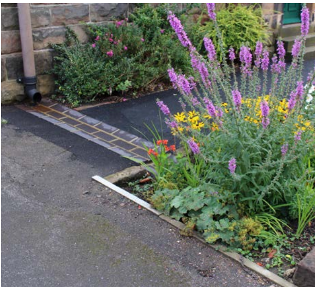
Image above: A retrofit downpipe shoe and brick channel into a rain garden.
