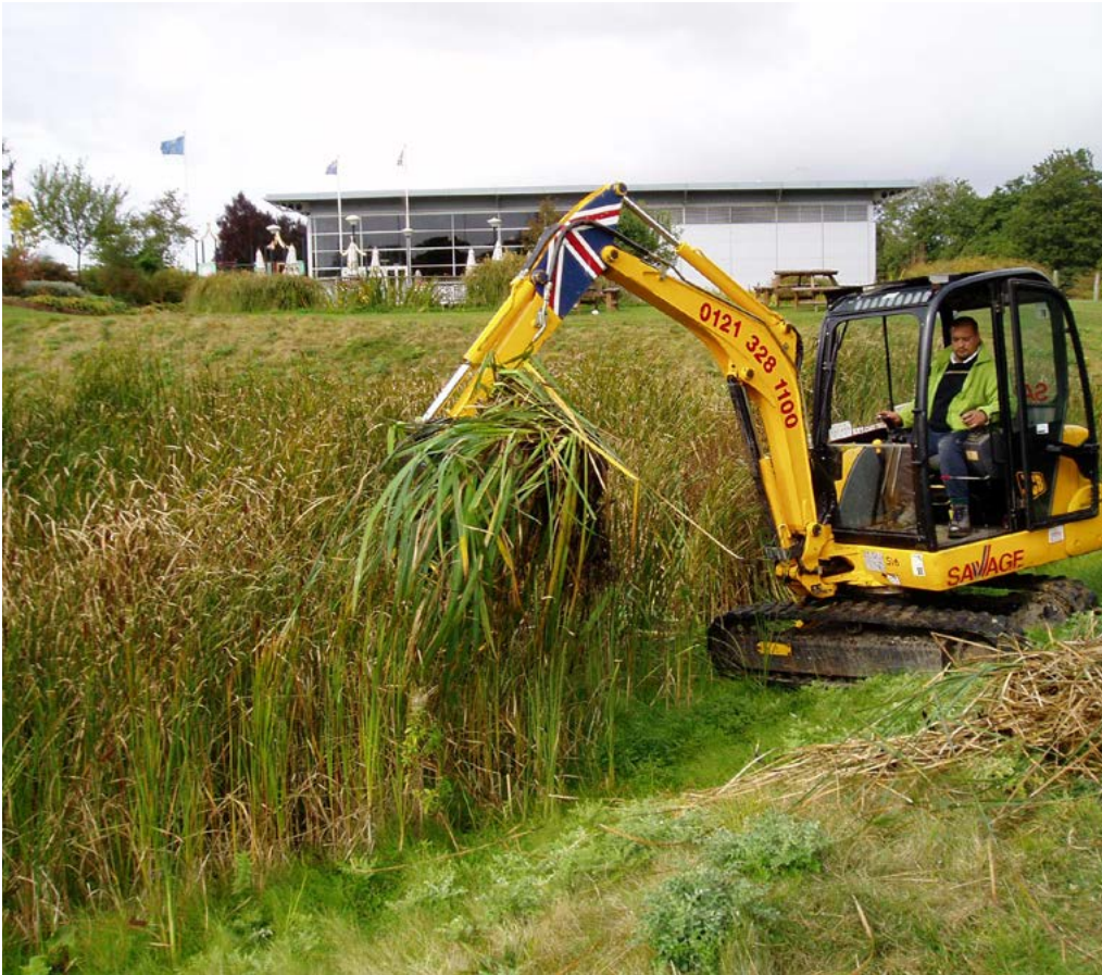
Image above: A light tracked excavator removes aquatic vegetation to de-water next to the wetland, before moving to a wildlife pile
