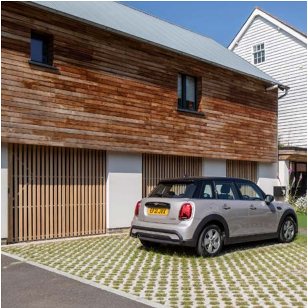
Image above: Void Structured Concrete paving - Cannock Mill, Colchester
