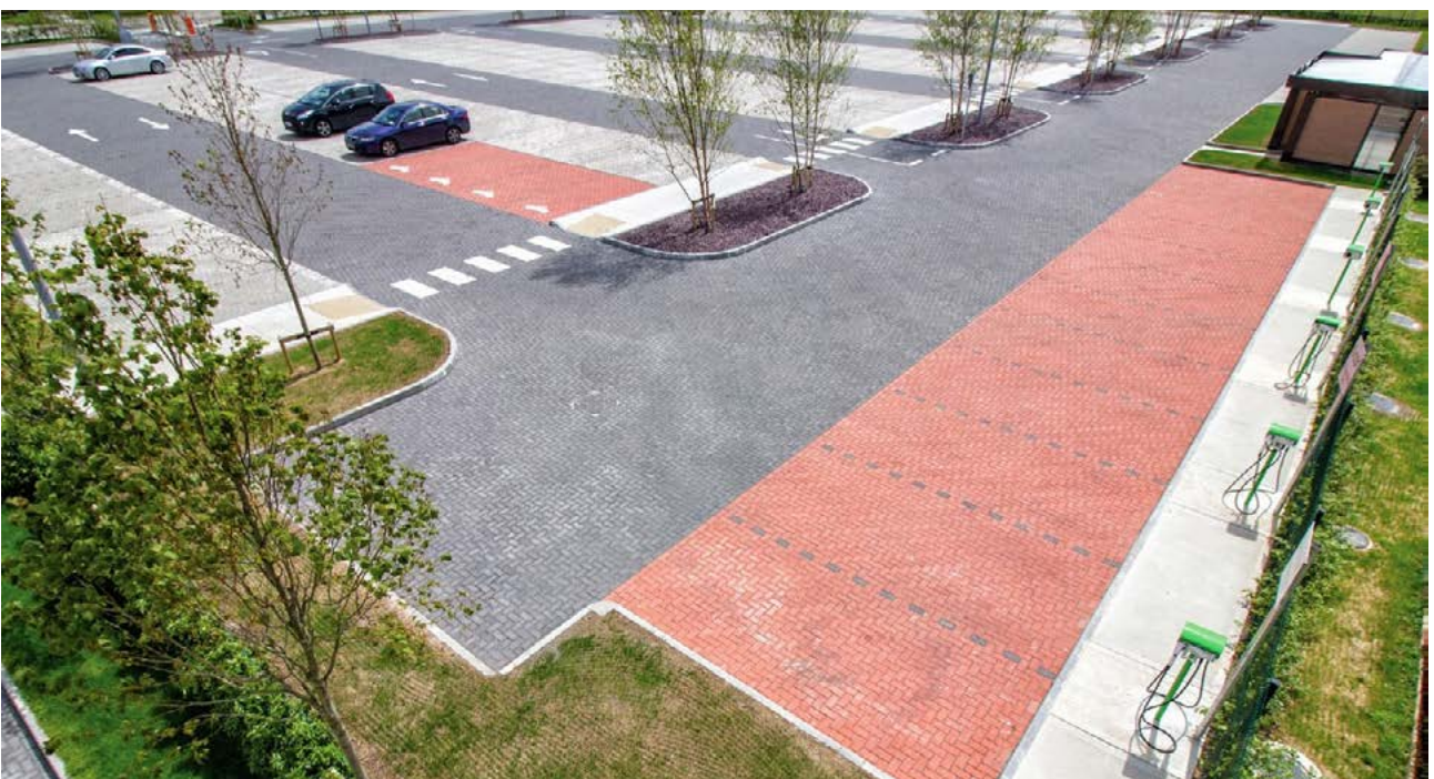
Image below: Post completion
