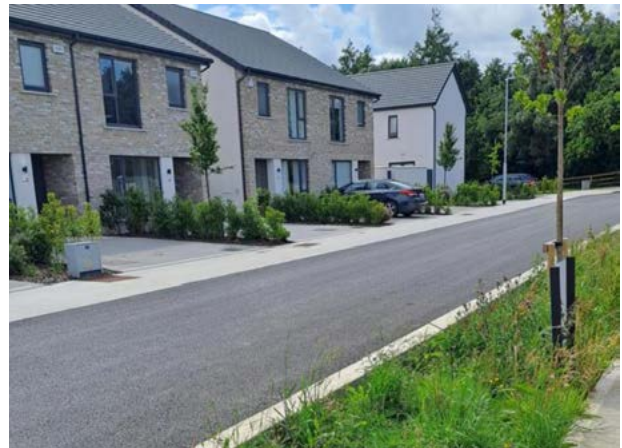
Image above: Collection of rainfall runoff through openings in kerb into a linear rain garden. Residential development, Leixlip
