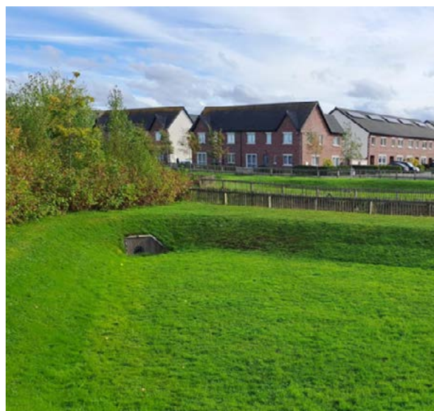
Image above: Detention Basin in public open space - Elsmore Naas
