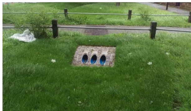
Image above: Concrete pipe surround has been used here to provide minimal cover for a driveway crossing
