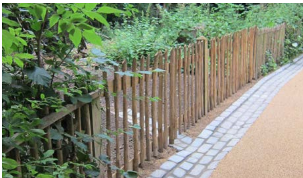
Image above: A granite sett channel collecting and conveying runoff
