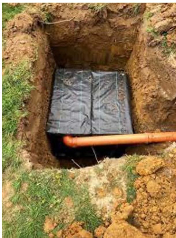
Image above: Example soakaway feature during construction
